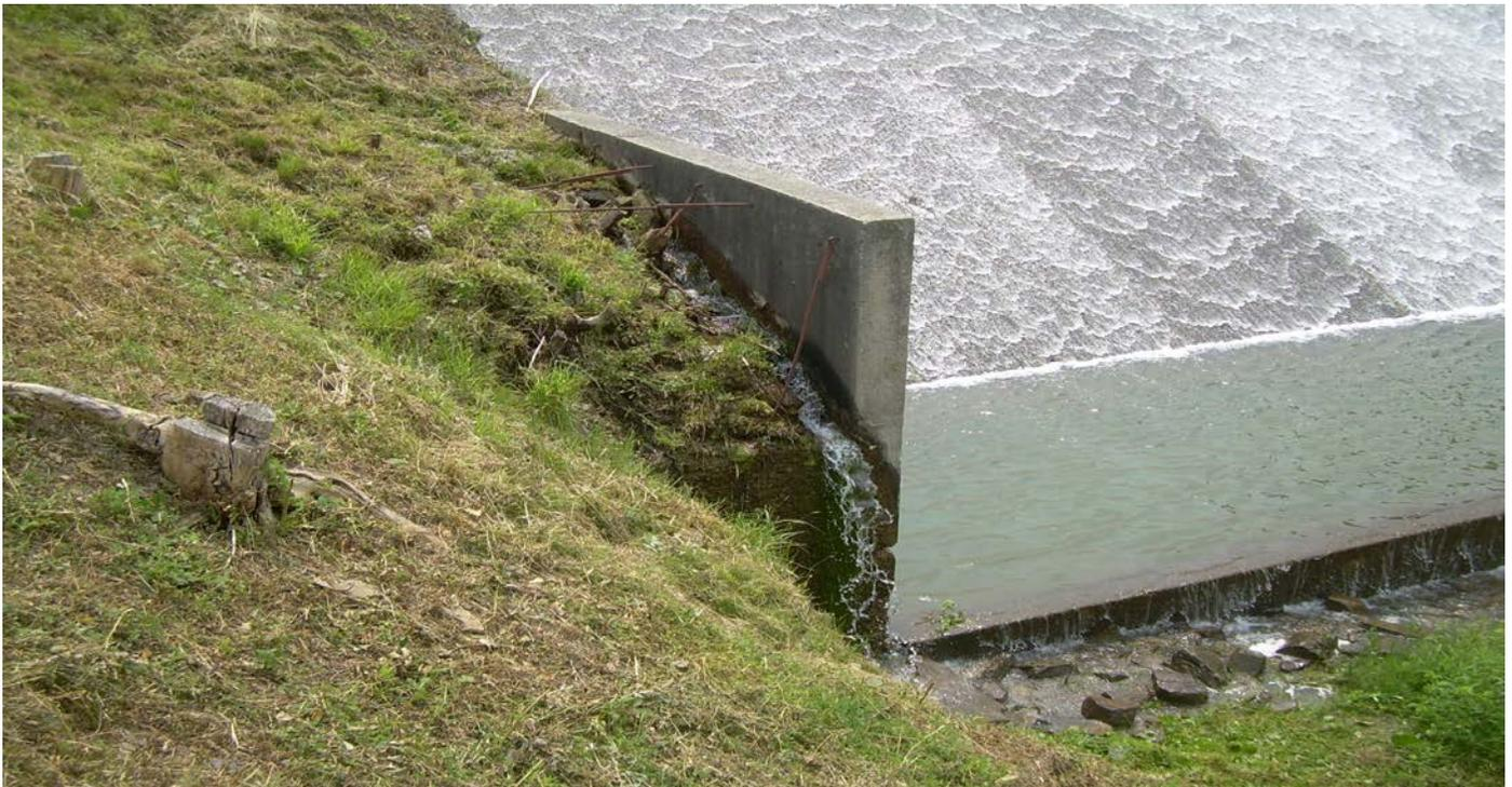
Recently there have been reports of a “leak” near the bottom of the spillway. Looking at the spillway, you may notice water running near the left wing wall. This is nothing new. Regardless, based on
